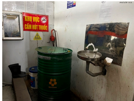
28. Eye-wash facility at chemical storage.jpg
